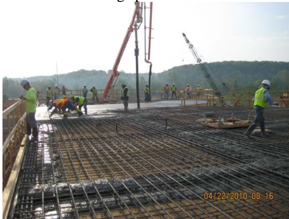
Placing concrete for Process Train decks
