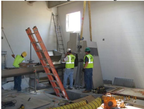
Setting screen unit in Screen Bldg
