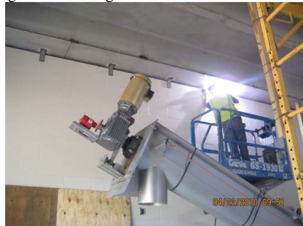
Welding wall closure piece in Screen Bldg.
