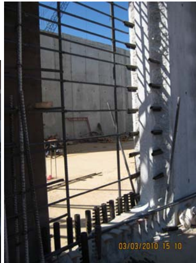
Mechanical splices at Process Train wall 74
