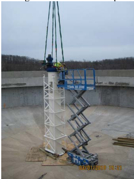
Beginning installation of Clarifier 62 equipment.
