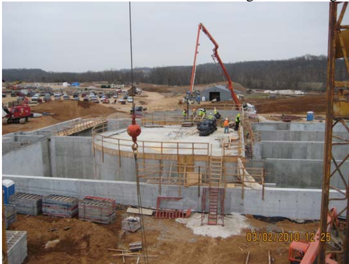
North deck Process Train 42 concrete placement
